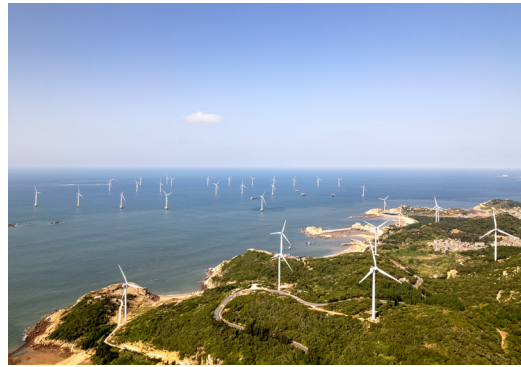
A bird's-eye view of a wind power plant in Fuzhou, Fujian Province, China (Getty Images)
